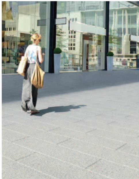
Example of good quality concrete paving slab
